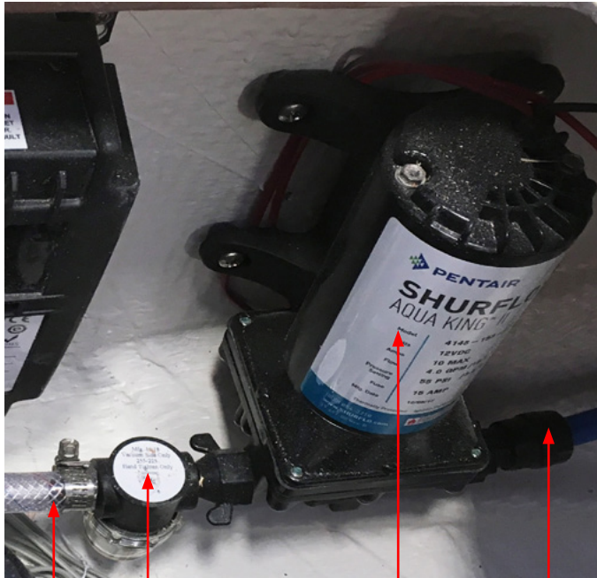
FILL HOSE FILTER/ STRAINER PUMP FEED HOSE
