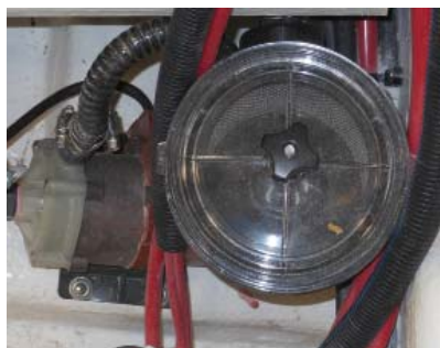
TYPICAL A/C SEAWATER STRAINER/BASKET
