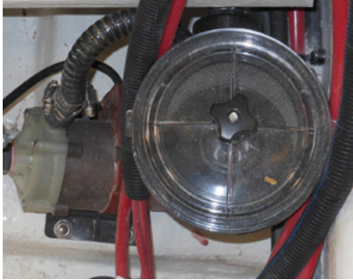
TYPICAL A/C SEAWATER STRAINER/BASKET
