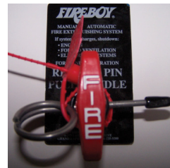
Typical Manual Discharge Pin For Automatic Fire Extinguisher
