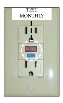
The GFIC (Ground Fault Interrupter Circuit, GFIC abbreviated) outlets should be tested monthly. To test the unit, depress the reset button. Then press the test button. The reset button should pop out.
