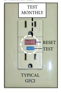
The GFCI is programed to protect a person from line to ground shock hazards which could occur from various electrical devices operating off of the device or receptacles down stream. It does not prevent line to ground electric shock, but does cut down the exposure time to a fraction of a second before the device trips. It does not protect people against
