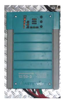
The yacht battery charger features 50 amp output and universal voltage for 3 battery circuits. This means that the battery charger will operate from 95 volts through 277 volts either at 50 or 60 Hz. This is helpful on docks that carry lower voltage. The new electronic battery chargers are "smart". They will charge the batteries in 3 stages; bulk, absorption, and float formats. The charger is
