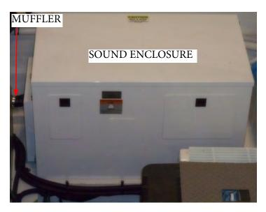
The generator features a sound enclosure which reduces noise and enables quick access for most inspections, troubleshooting and routine maintenance.
