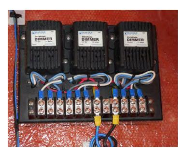
The dimmer switch panel controls the salon dimming switches on the 3 gang panel at the port side of the steps at the atrium (steps to lower level). There is no normal maintenance to this panel. It is located just below the 3 gang dimmer light switches at the stairway.
