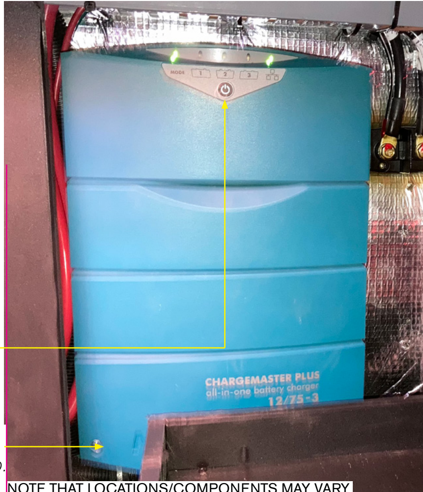
BATTERY CHARGER- (NOTE THAT OPTIONAL 75 AMP O/B CHARGER SHOWN; STD. CHARGER AMPERAGE IS 50)
