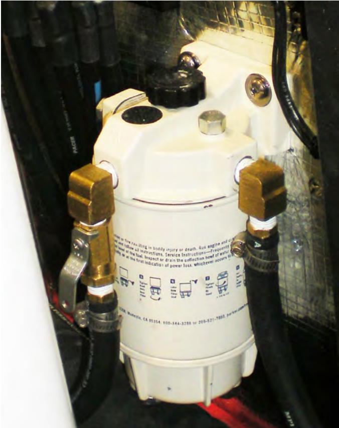
DIESEL GEN-SET PRIMARY IN-LINE WATER SEPARATOR FILTER
