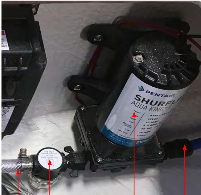
FILLHOSE FILTER/ STRAINER PUMP FEED HOSE
