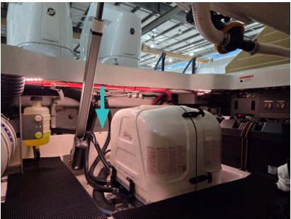
Aft bilge pump
